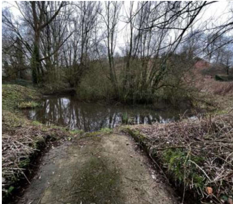
Figure 28 Flood relief pond opposite Hadspen Valley Farm, constructed 1984
